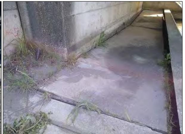
③ 橋梁基礎の沈下・噴砂
